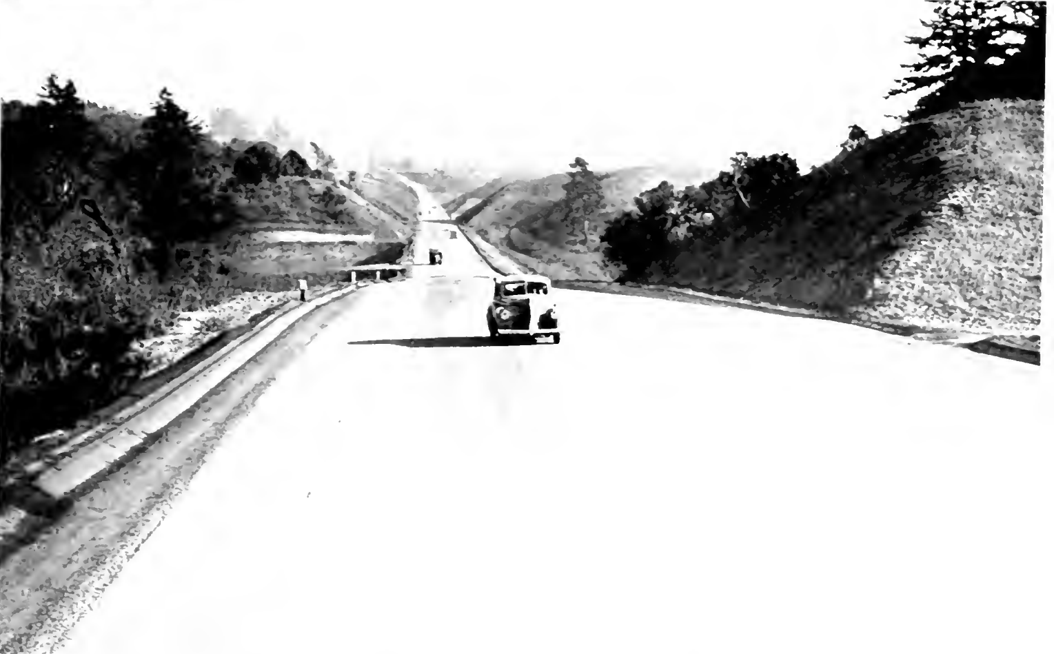
Two views of three-lane highway between Watsonville and Red Bluff Junction, where the old two-lane road had an acute left-hand curve that caused congestion in Pajaro Valley. Highway ultimately will extend to Santa Cruz.
